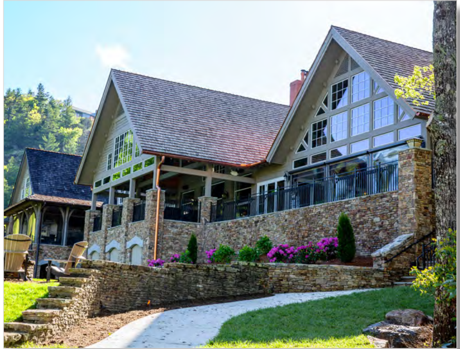
IMAGE ABOVE: EXTERIOR VIEW AFTER CONSTRUCTION.
