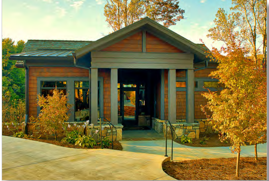
IMAGE ABOVE: EXTERIOR VIEW OF CONSTRUCTION
