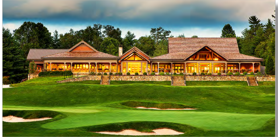
IMAGE ABOVE: EXTERIOR VIEW OF CONSTRUCTION.
